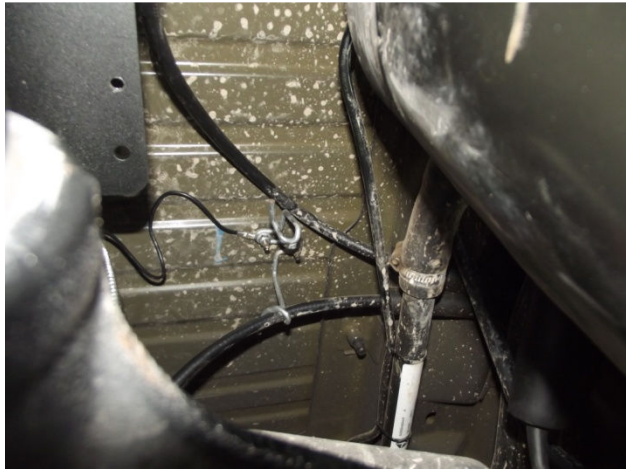
Photo 7 – Emergency brake cable support
